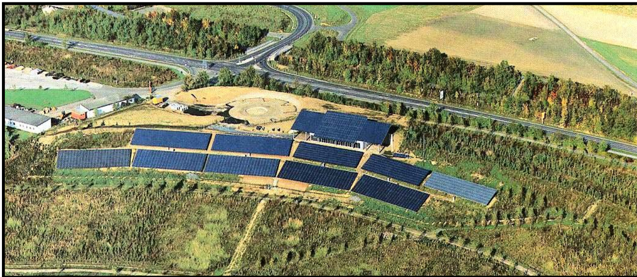
PV Neurather See (Alemanha) 360kWp
