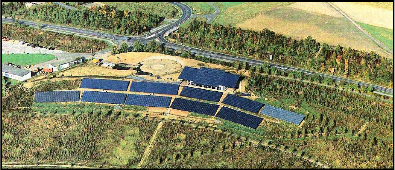
PV Neurather See (Alemanha) 360kWp
