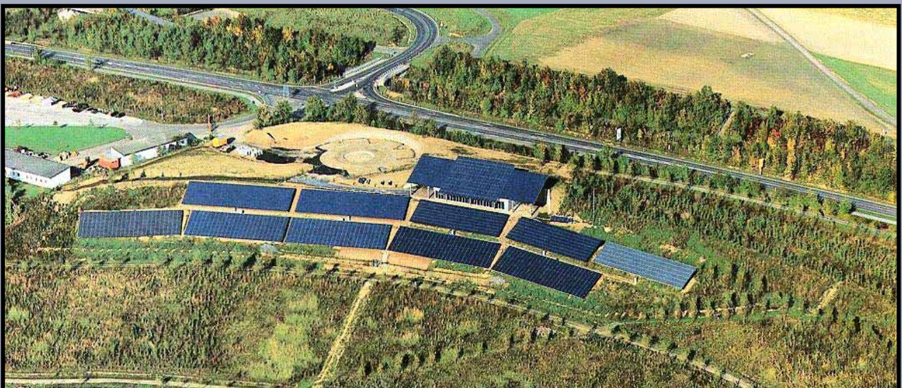
PV Neurather See (Alemanha) 360kWp
