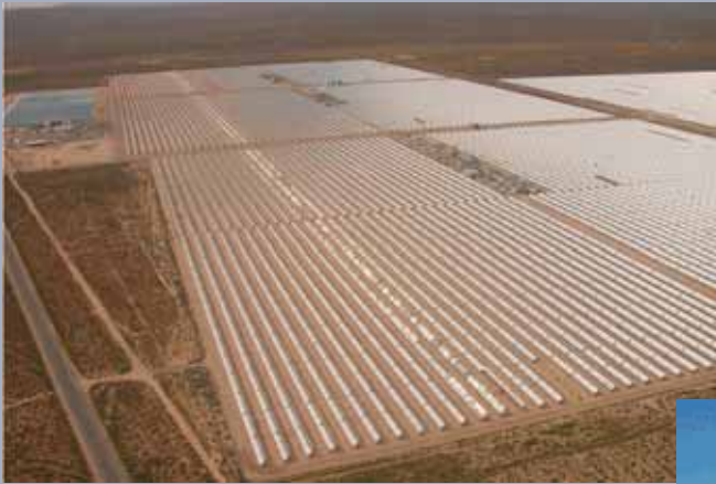
SEGS, Kramer Junction, California, USA 354 MW.
