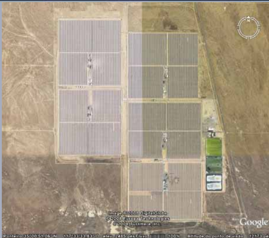
SEGS, Kramer Junction, California, USA – 354 MW; 2,3 km 2
